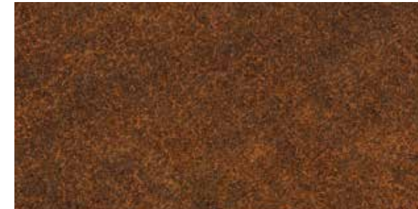
2. Appearance/shades of oxidized product after approximately 4/6 months from its installation.
